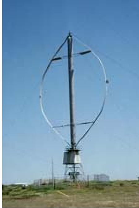
Figura 2.9 – Turbina Darrieus [Danish Assoc].
